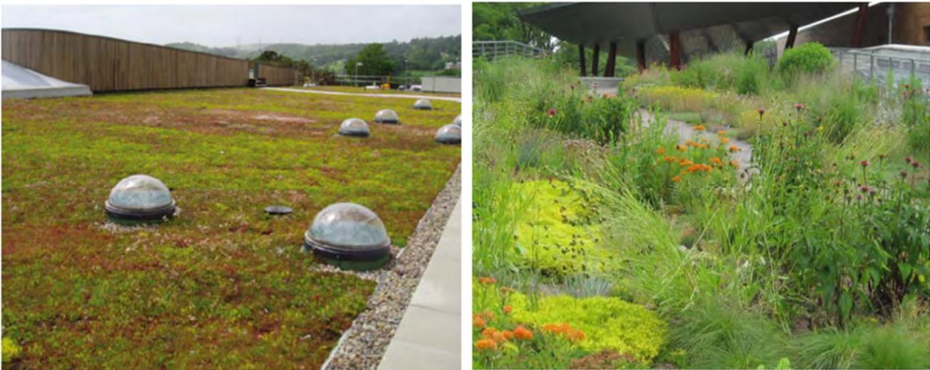
*Figure 5.2. Example of extensive green roof (left) and intensive green roof (right)<sup>162</sup>*
